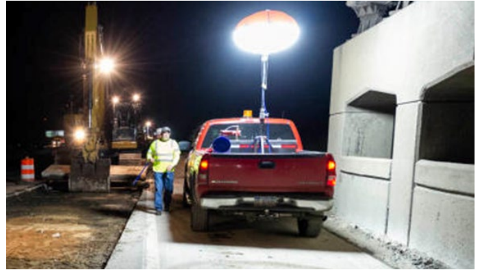
Figure 4. Nighttime Work Zone Using Balloon Lighting (Source: Michigan DOT)
