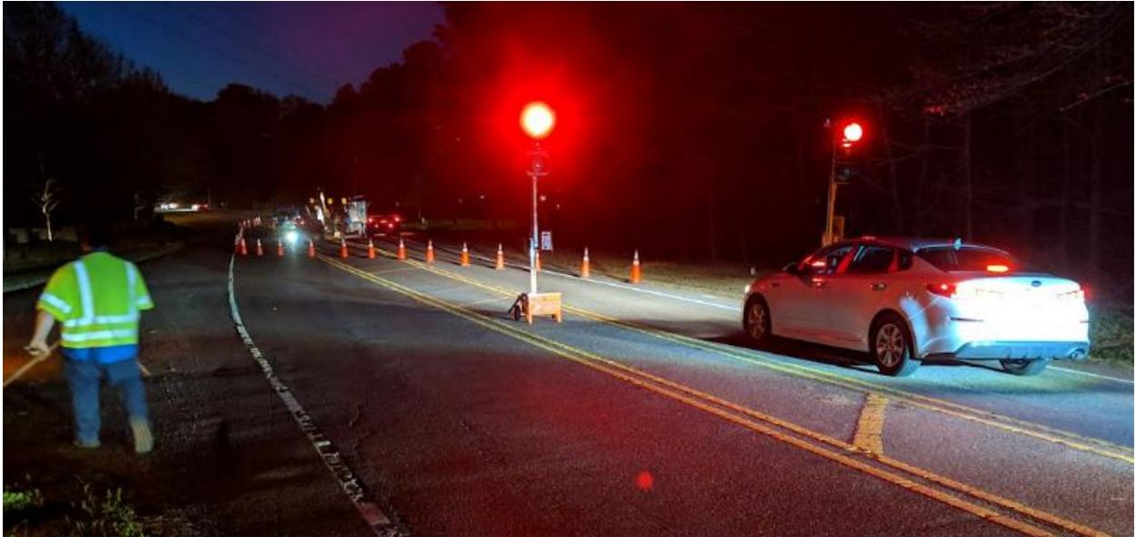
Figure 7. Pedestal-Mounted Portable Traffic Signals (Image: Branz Technologies)
