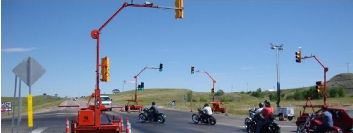
Figure 6. Temporary Signalized Intersection in Sturgis, S.D. Using PTS (image: Street Smart Rentals)
