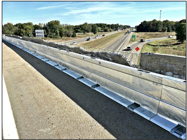
Figure 4. Positive Protection on a Bridge Segment Using Temporary Steel Barrier (Image Courtesy of Hill and Smith, Inc.)
