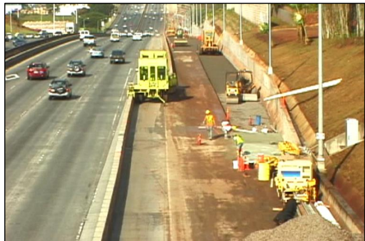
Figure 3. Moveable Concrete Barrier Expanding Work Space Access (Image Courtesy Barrier Systems, Inc.)
