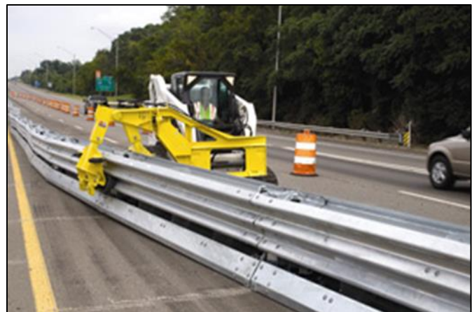
Figure 5. Moveable Steel Barrier Reconfigured Using a Front Loader Attachment (Image Courtesy of ATSSA)
