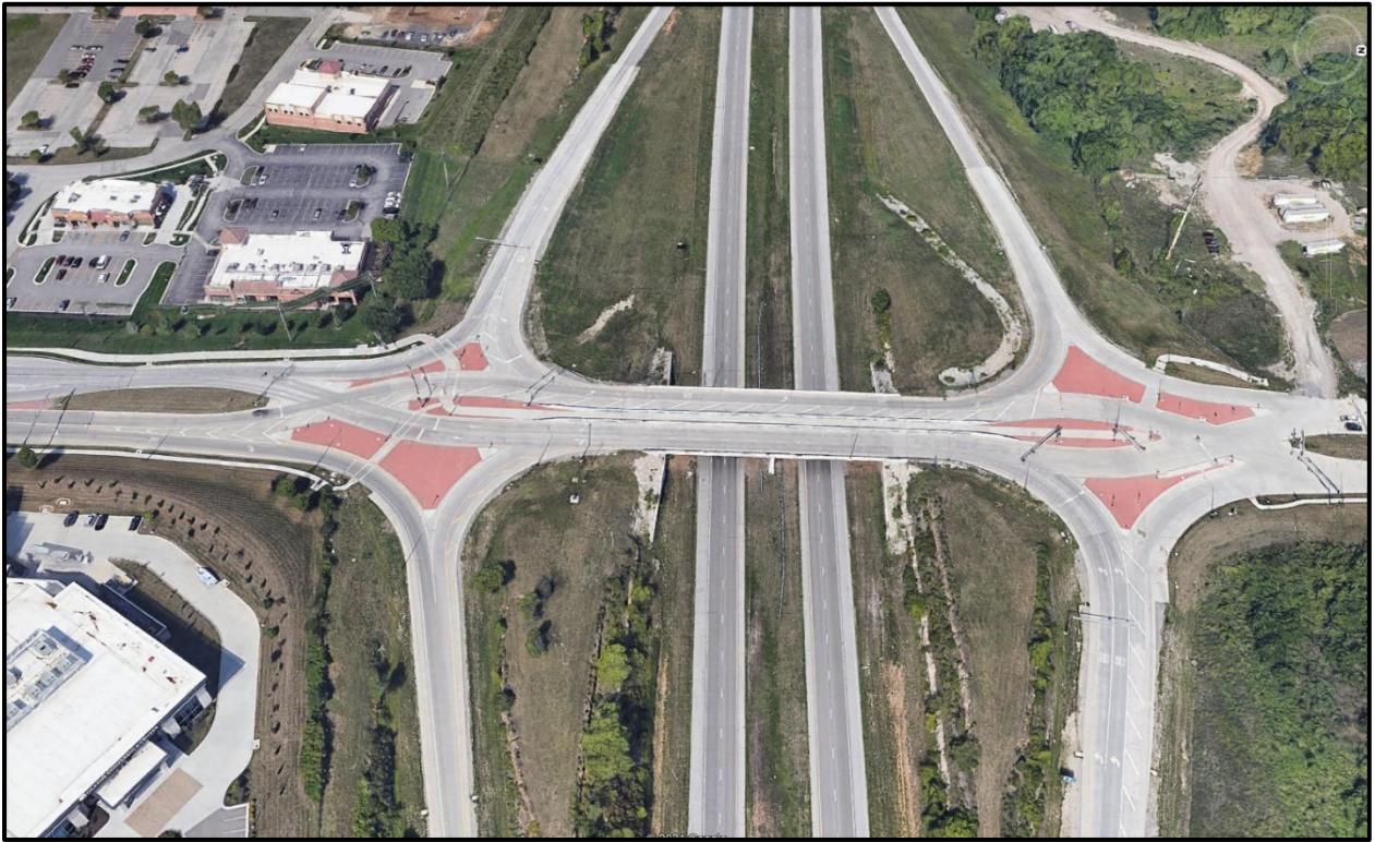
Figure 23. Aerial view of a DDI (K-10 and Ridgeview Road, Olathe/Lenexa, Kansas) (Source: Google Maps, 2022)
