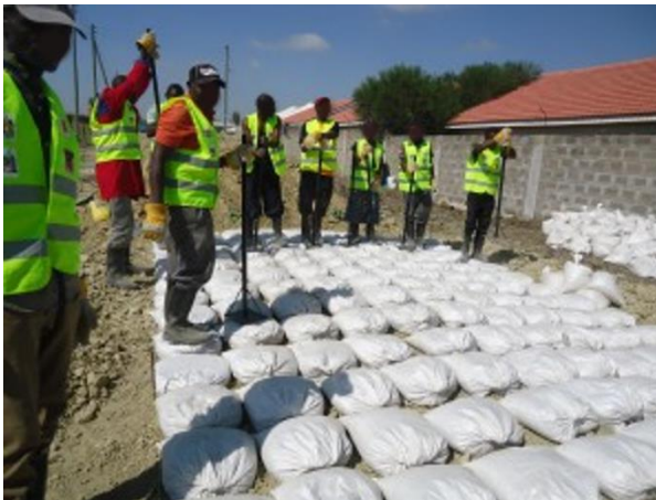
(c) Placing and hand-tamping upper layer
