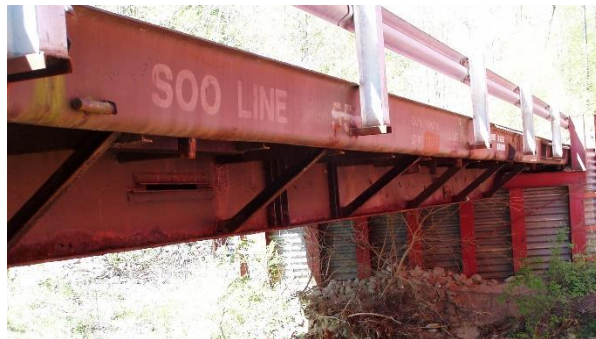
Figure 109. Railroad flatcar converted to a temporary bridge.
