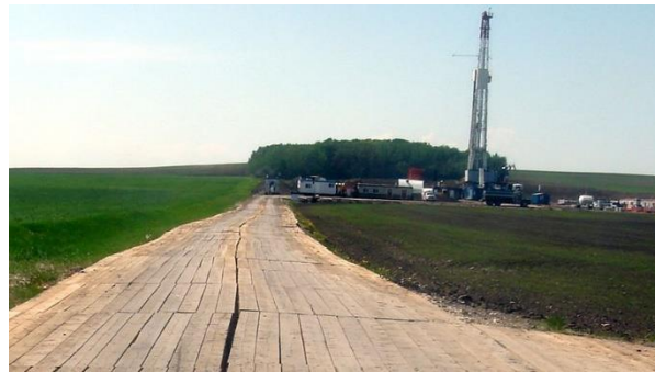
Figure 29. Timber plank road built over unstable soil.
