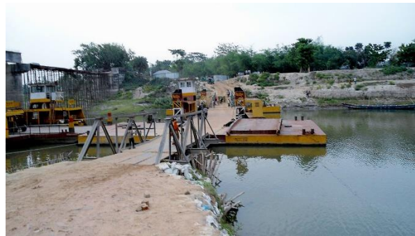
Figure 2. Floating bridge for a temporary river crossing and its approach road.
