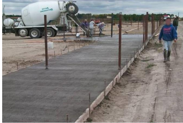
S. Birchall / North Dakota State University Figure 37. Flatwork paving with CLSM.
