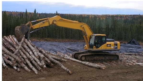
Figure 30. Placing corduroy over unstable soil with a tracked excavator.
