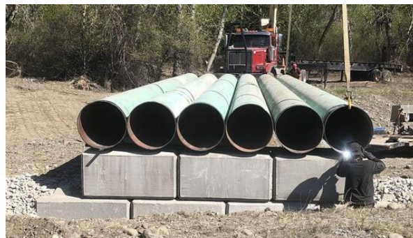
Figure 97. Steel pipe bridge under construction.
