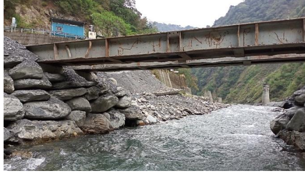
Figure 108. Temporary bridge under construction featuring salvaged steel beams.
