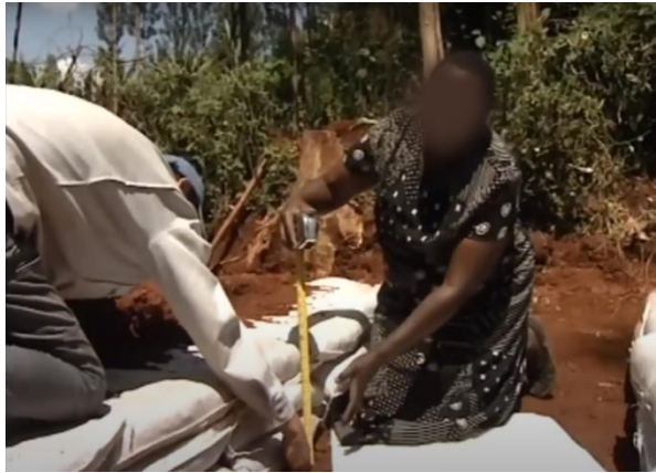
(b) Checking wall height after placing the third layer of bags.
