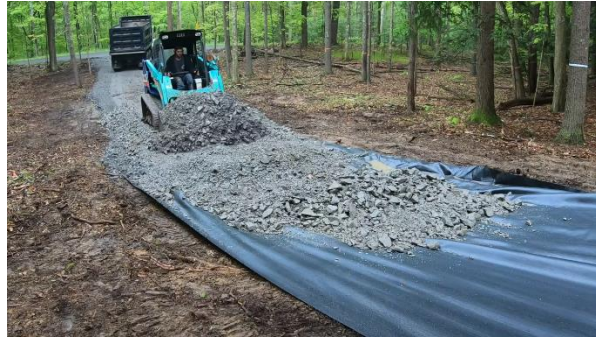
Figure 13. If available, geotextile can help stabilize temporary roads by spreading wheel loads across the underlying soil more evenly.
