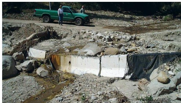
Figure 60. Temporary unvented ford built from Jersey barriers and rock backfill in response to a wildfire (California, 2004).
