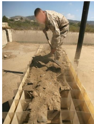
United States Marine Corps Figure 38. Geocell grid helps stabilize gravel, sand, and soil by limiting lateral movement.
