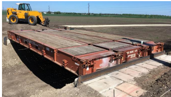
Figure 110. Flat racks (ISO folding end wall containers) have been used as bridges.
