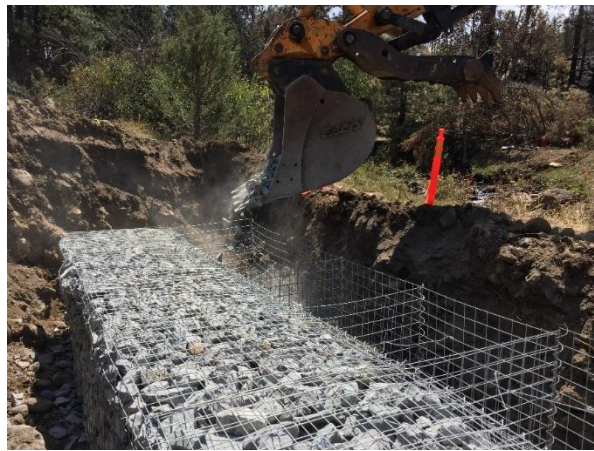
Figure 121. Preparation of gabion for use as a temporary bridge footing after a forest fire.
