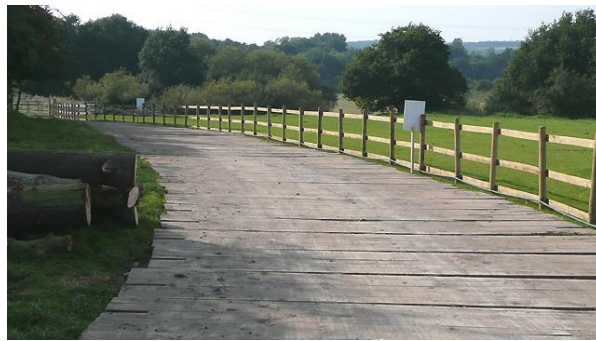
Figure 42. Temporary road assembled from prefabricated mats.
