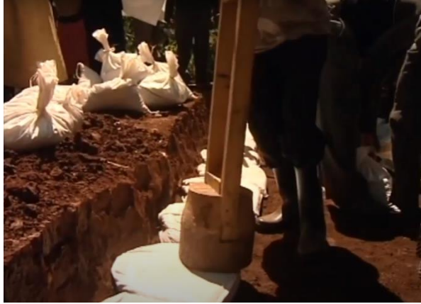
(a) Placing and compacting the first layer of aggregate bags to form the culvert wall.
