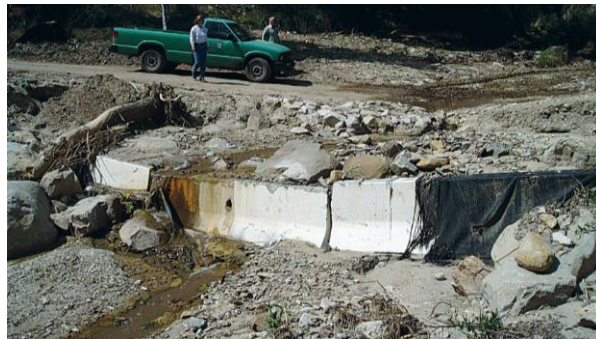
Figure 75. Temporary low-water crossing built from Jersey barriers and rock backfill in response to a wildfire.
