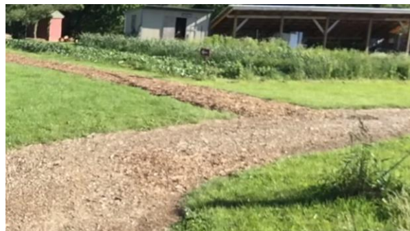
Figure 27. Road surfaced with wood chips after one year of use by light commercial traffic.
