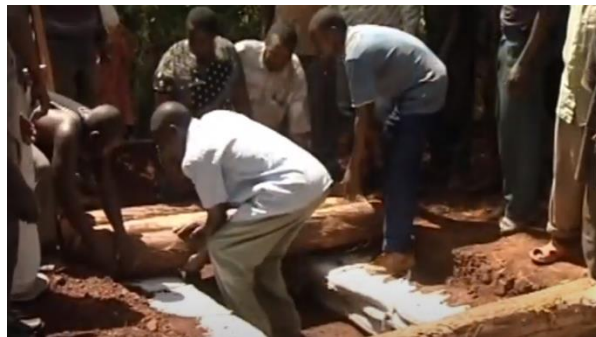
Figure 15. Hand construction of a box culvert using timbers and compacted bags of gravel.
