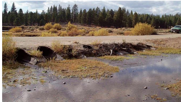
Figure 59. Upstream side of a vented ford.
