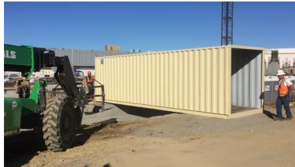
Figure 87. Shipping container being repurposed as a temporary pedestrian bridge.
