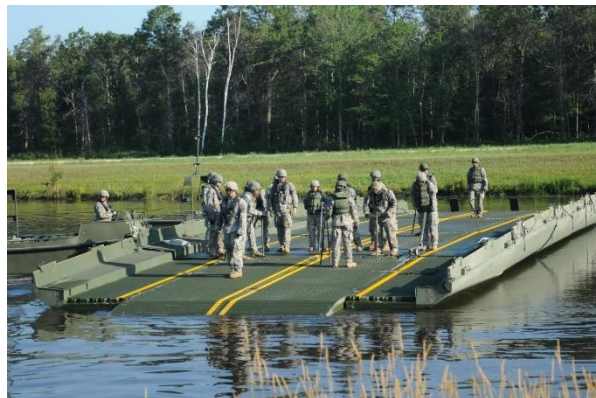
Figure 118. Deployment of an Improved Float Bridge (Ribbon).
