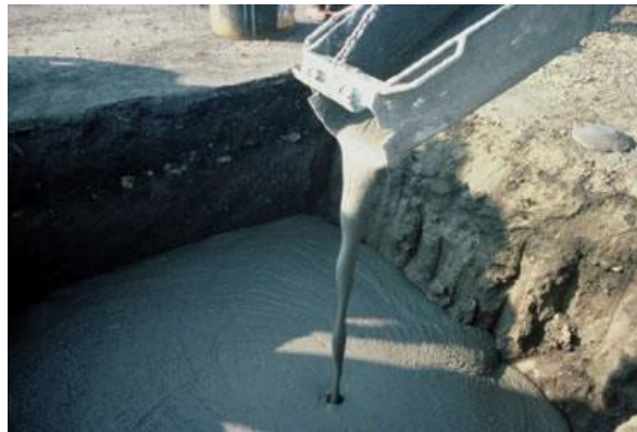
Figure 36. Discharging CLSM from a mixer truck.
