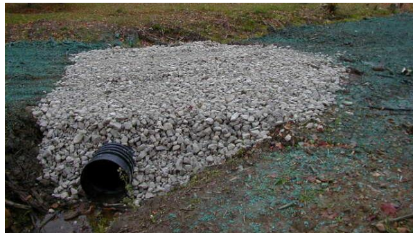
Figure 14. Temporary culvert backfilled with gravel.
