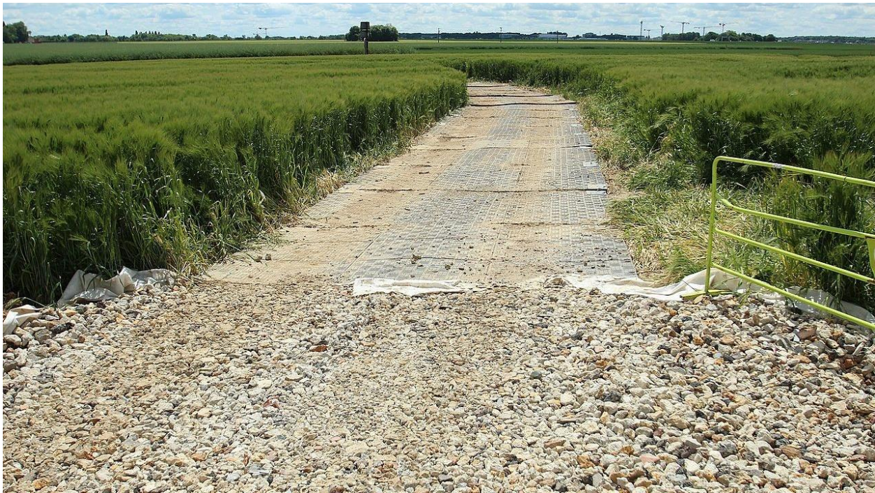
Figure 26. Gravel over geotextile (foreground) and plastic mats (background) used to build a temporary road.
