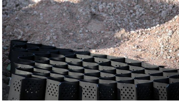
Figure 63. Geocells can reduce erosion of gravel-surfaced low-water crossings.
