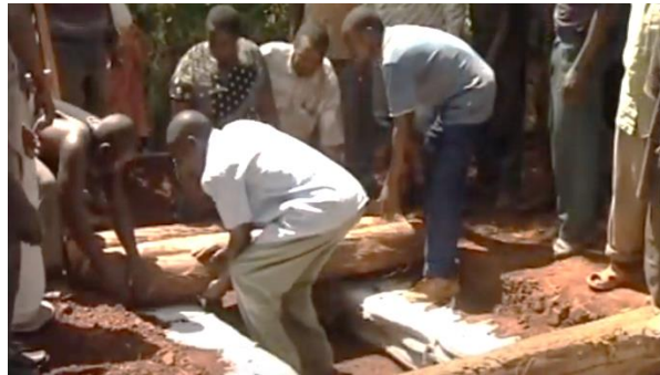
Japan International Cooperation Agency / https://www.youtube.com/watch?app=desktop&v=zcG7cdKXKxU Figure 77. Hand construction of a box culvert using timbers and compacted bags of gravel.
