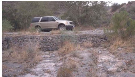
Figure 57. Gabion ford on an intermittent waterway.
