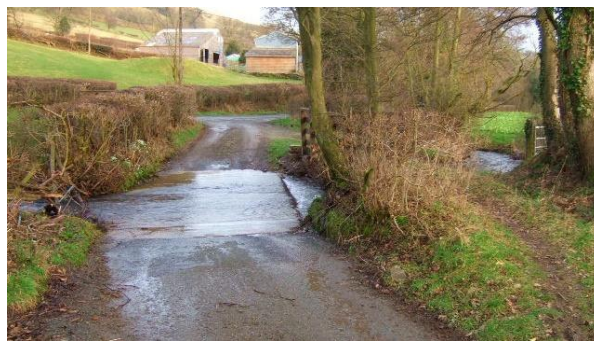
Figure 18. Low-water crossings are an expedient solution for crossing small waterways.
