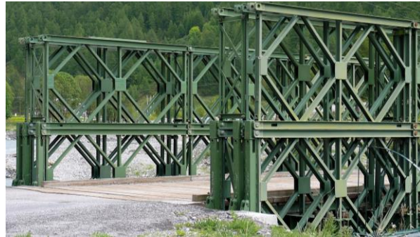
Figure 100. Bailey bridge with horizontally tripled and vertically doubled panels.
