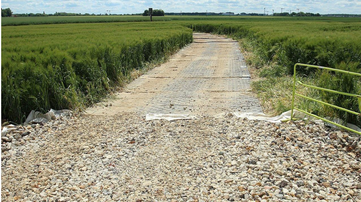
Figure 33. Gravel over geotextile (foreground) and plastic mats (background) used to build a temporary road.
