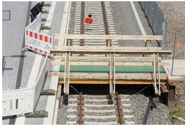
Figure 82. Temporary pedestrian bridge fabricated from lumber.
