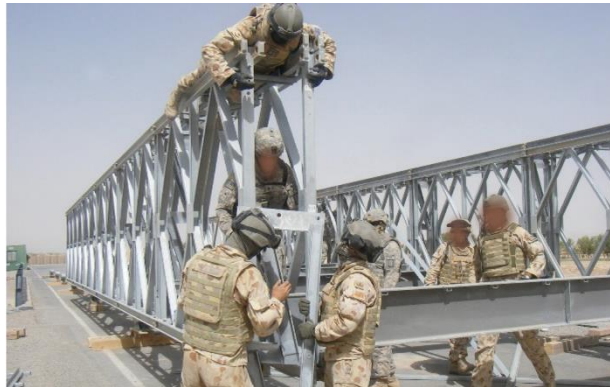
Figure 103. Assembling a Mabey bridge.
