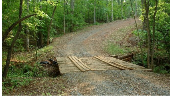
Figure 19. Plank surfacing is sometimes used for temporary bridges.
