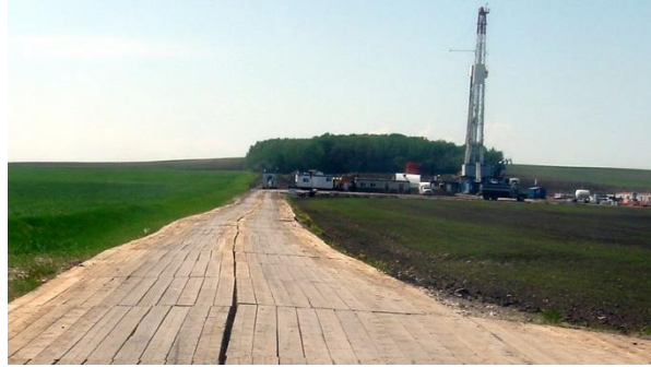
Figure 41. Timber plank road built over unstable soil to allow heavy equipment to reach a drilling site.
