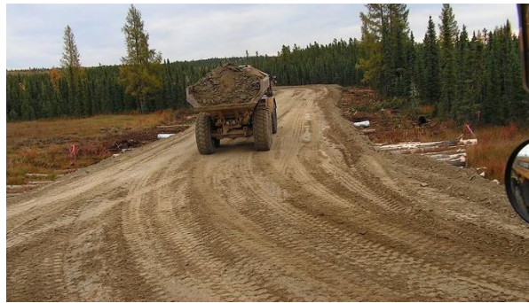
Figure 44. Corduroy road after backfilling with earth.
