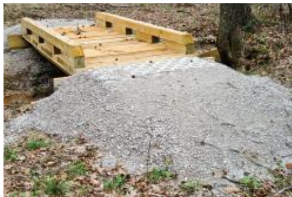
Figure 83. Short-span timber bridge for pedestrians and ATVs.
