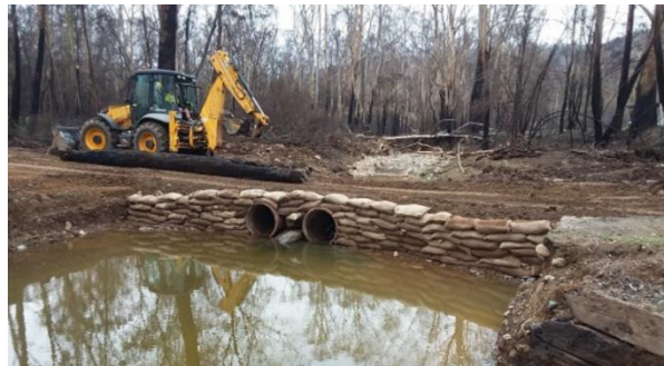
Eurobodalla Shire Council Figure 78. Temporary culvert with sandbag headwalls, used to bypass a fire-damaged bridge.
