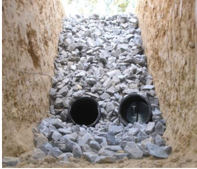
Figure 16. Trench drains (trenches backfilled with gravel) can be installed to manage stormwater.
