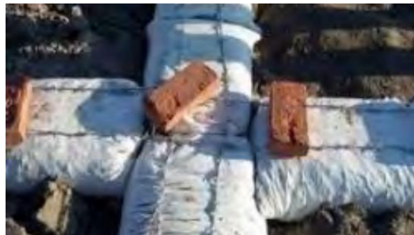
(b) For stability, the bottom of a bagged-aggregate retaining wall should extend out farther than the top (battered wall).
