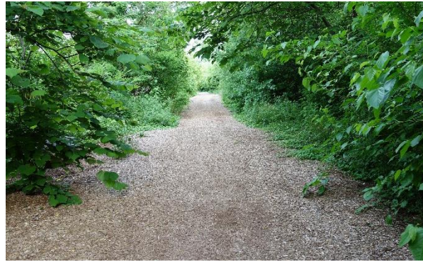
Figure 34. Trail surfaced with wood chips, New York City.
