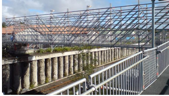
Figure 86. Temporary pedestrian bridge assembled from scaffolding components.
