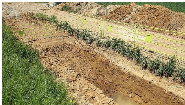
Figure 12. If time and resources allow, vegetation and topsoil can be removed to improve the durability of a temporary road.
