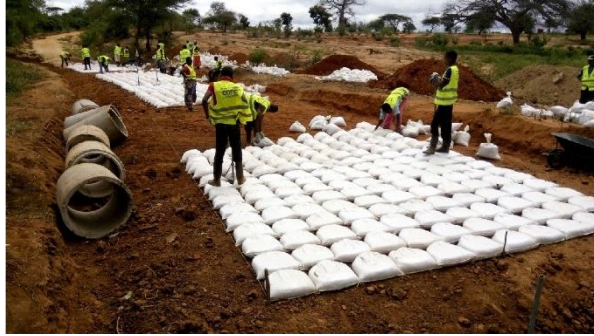
(a) Placing lower layer of a bagged-aggregate road
