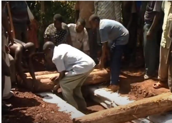
(c) Heavy timbers span the channel.
