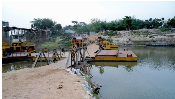
Figure 89. Floating bridge for a temporary river crossing and its approach road.
