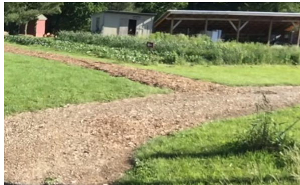
Figure 35. Road surfaced with wood chips after one year of use by light commercial traffic.
