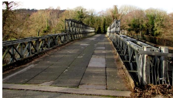
Figure 101. Bailey bridge with horizontally and vertically doubled side panels; semipermanent application.
