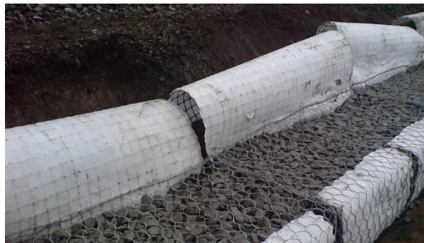
Figure 21. Gabions (rock-filled wire baskets) can be used to stabilize the toe of a steep side slope.
