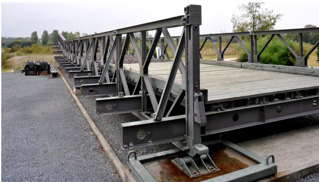
Figure 99. Bailey bridge display, illustrating the side panels, transoms, stringers, decking, and roller footings, with a launching nose visible at the far left.
