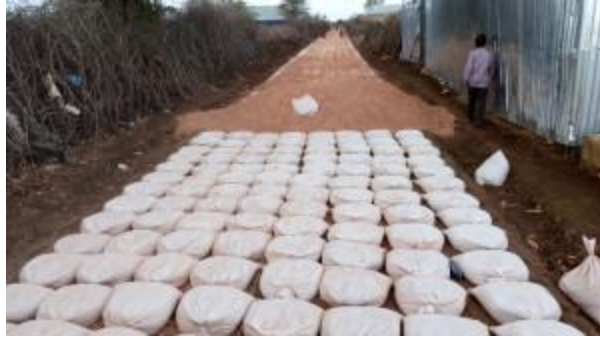
Figure 28. Bagging gravel, sand, or soil improves its stability, allowing a strong road to be built without heavy equipment. The bags can be stacked to build box culverts and retaining walls.
