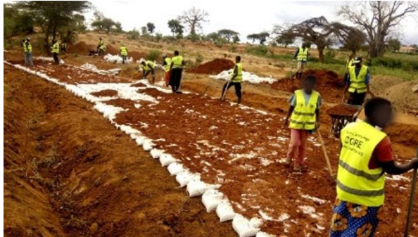
(b) Spreading gravel interlayer
