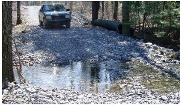
Figure 17. Gravel pads are sometimes adequate for crossing small waterways.
