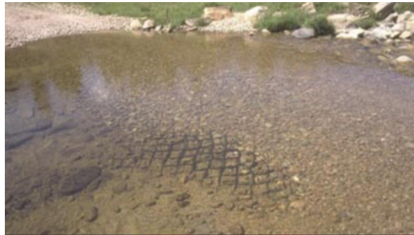
Figure 64. Geocells partially exposed by traffic and water movement.
