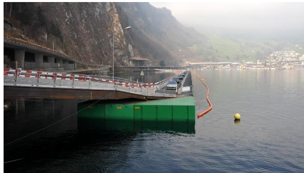
Figure 20. Pontoon bridges have long been used for temporary crossings of large waterways.
