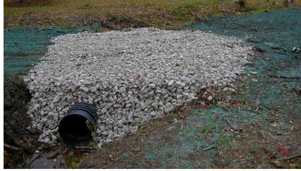
© Massachusetts Department of Environmental Protection Figure 76. Temporary culvert backfilled with gravel.
