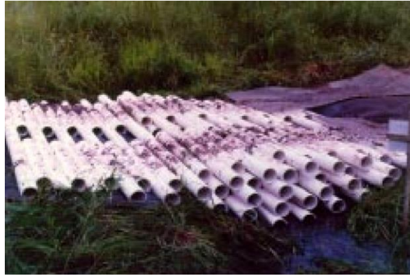
Figure 81. PVC pipe bundle crossing for a ditch or small waterway.
