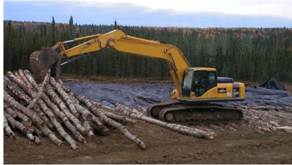
Figure 43. Placing corduroy over unstable soil with a tracked excavator.
