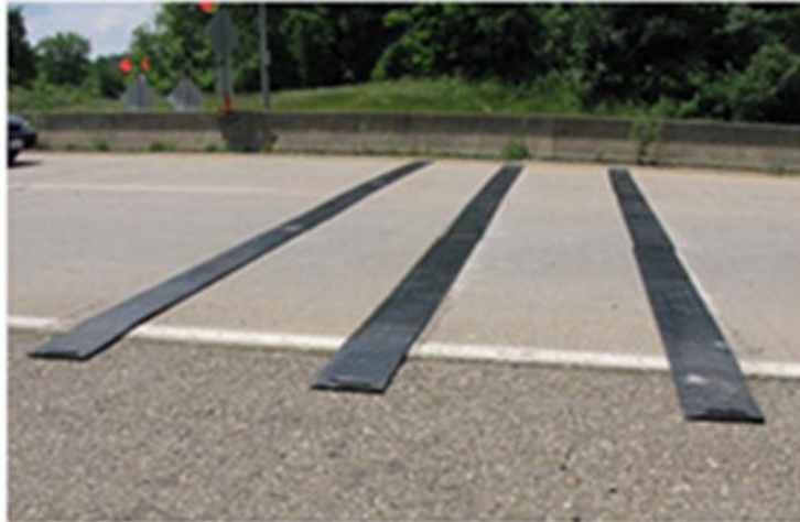
Figure 5.4. Portable rumble strips
