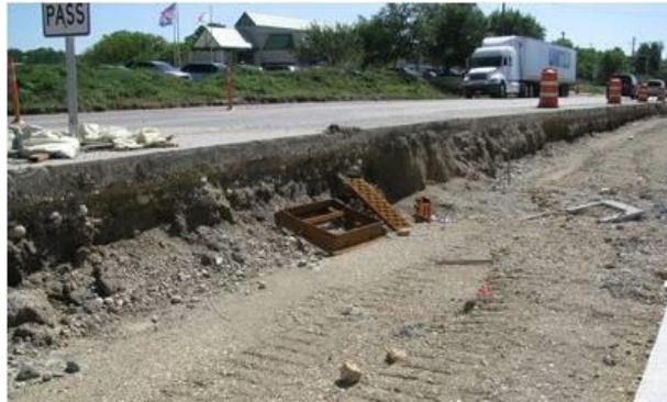
Figure 2. Abrupt pavement edge drops create the potential for serious crashes. Photo: Wisconsin DOT
