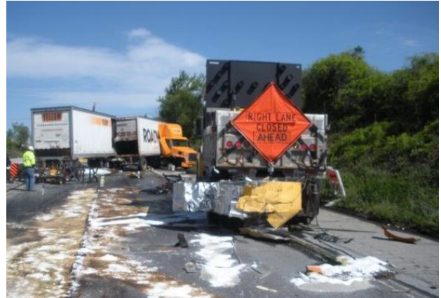
Figure 19. Spreading absorbent material to soak up spilled diesel fuel. Photo: Pennsylvania DOT
