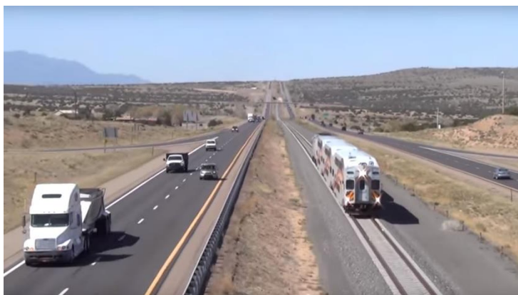
Figure 12. New Mexico Rail Runner, a commuter train connecting Belen, Albuquerque and Santa Fe, operates partly in the median of I-25. Photo: Aaron Friedman/YouTube
