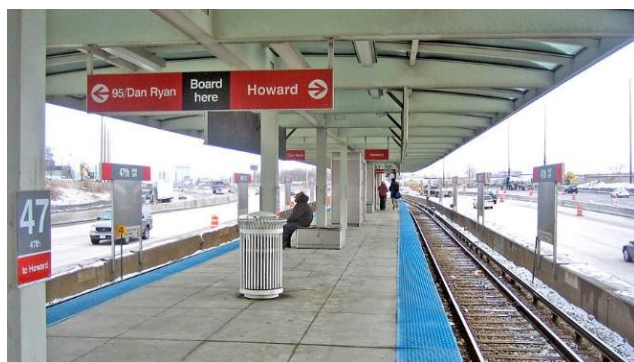
Figure 11. The Chicago Transit Authority's Red Line is one of several U.S. mass transit facilities located in freeway medians. An electrified third-rail is visible at the lower right. Photo: Graham Garfield/WikiMedia Commons
