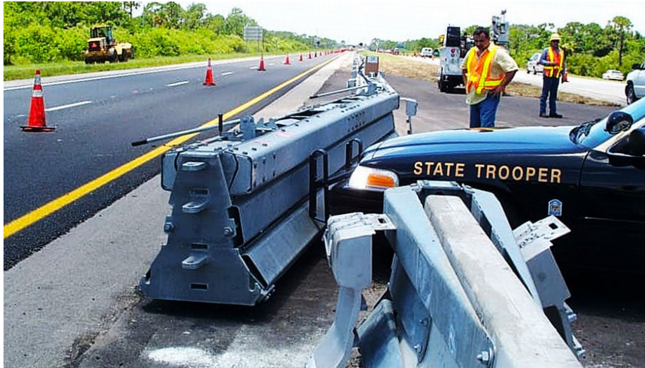
Figure 56. Barrier gates can facilitate access for emergency vehicles and delivery of heavy equipment to the jobsite.
