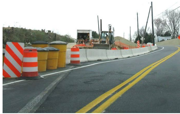
Figure 21. Temporary portable concrete barrier with sand-filled drums as an end treatment on a 2-lane rural highway project. Source: Wikimedia Commons/
