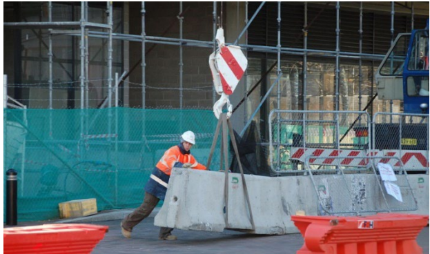
Figure 7. Barrier installation requires equipment, labor, and preparation. Source: Wikimedia Commons/BenAveling
