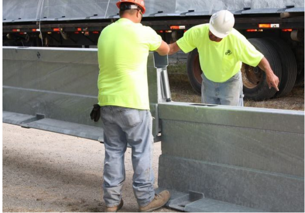
Figure 38. Installation of a steel barrier system.
