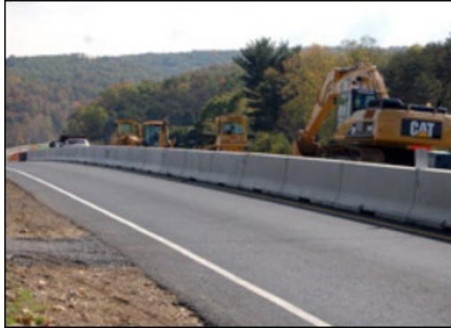
Figure 6. Positive protection for motorized traffic and shielding workers.
