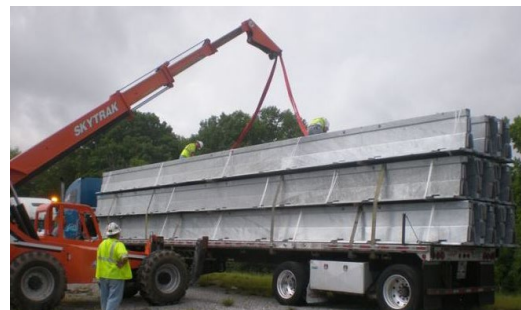
Figure 41. Unloading steel barrier segments using a rough-terrain forklift.
